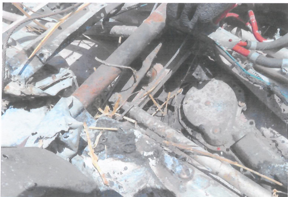
Photo 18: The transverse rods connecting the flaps
