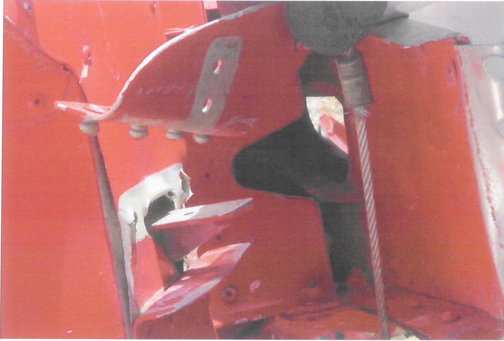
Photo 9: Detached elevator bracket lower surface
