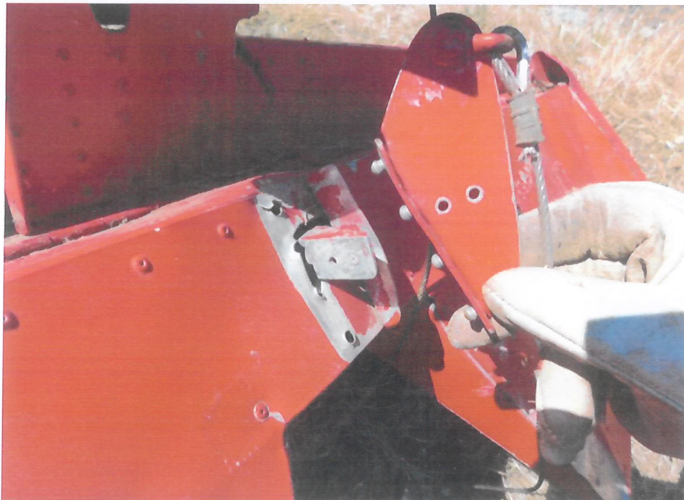
Photo 10: Elevator end connection lower surface
